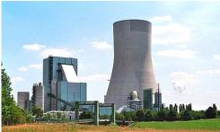
18. Many power plants cool their reactions with convective air flow through a hyperboliod tower. The shape increases air flow while minimizing construction
