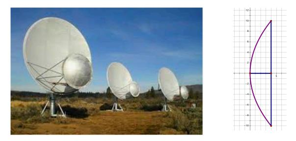
17. The SETI Institute (search for extra-terrestrial intelligence) began using the Allen Telescope Array (ATA-42) in 2016 to search for intelligence among radio waves. ATA-42 is a set of 42 radio receivers with parabolic dishes. Each dish conforms to the shape formed by revolving the equation  $y=5\sqrt{x}$  revolved about the x-axis from x=0 to x=4 ft.
